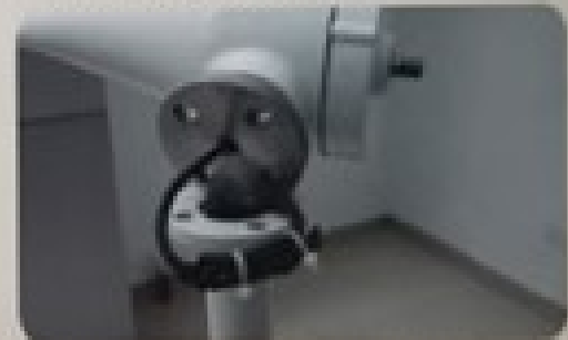
4. Connect 3 wires to transmission cables so that they are long enough to be pulled out from the bottom of tower.
